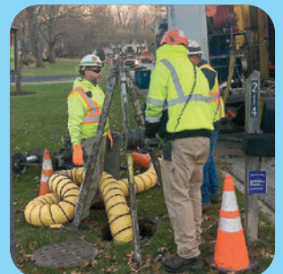
Adding lining to existing pipes to extend the life of the sanitary sewer pipes.
